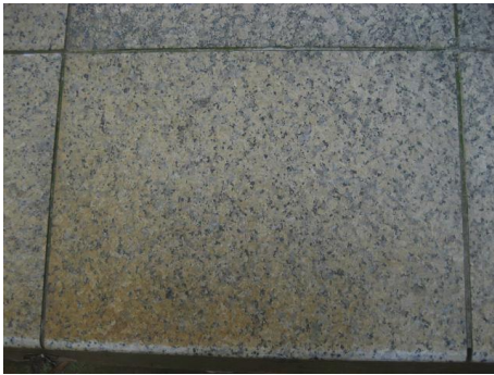
Before (Iron rust)
